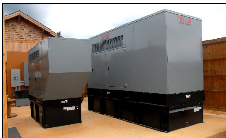
The models pictured above are the (left) TD100 and the (right) TD250. Both of these units are equipped with the sound attenuating option and the DGC2020 control panel.
